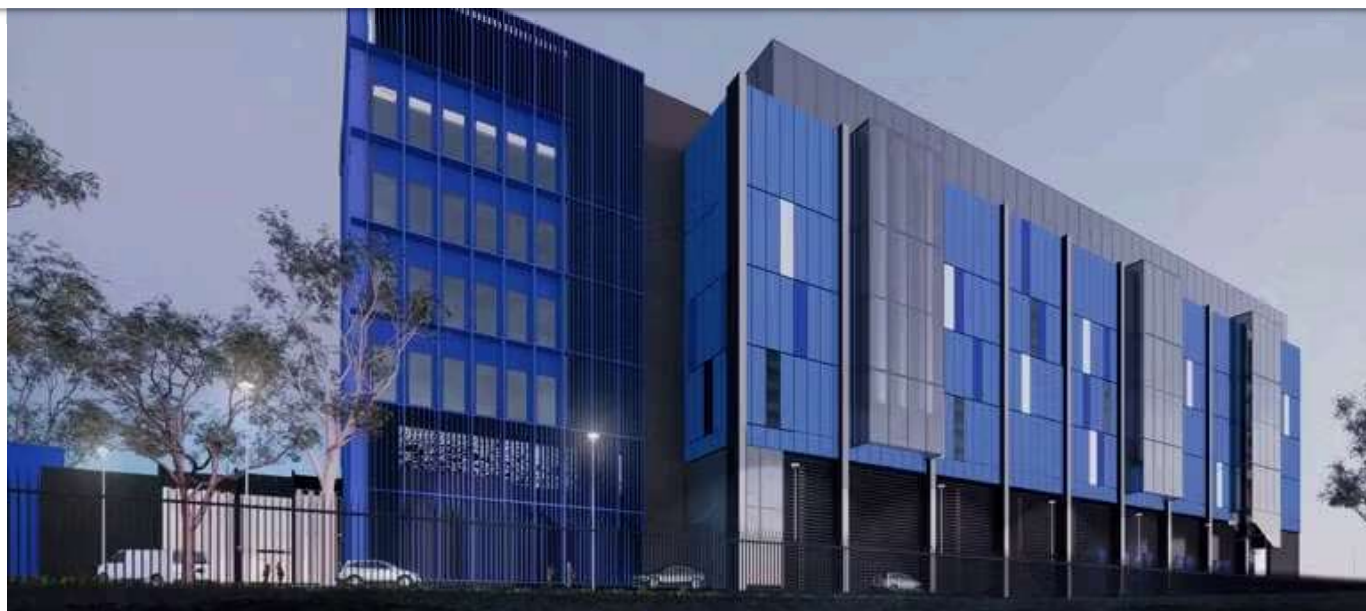
Macquarie Park Data Center Campus in Sydney, Australia
