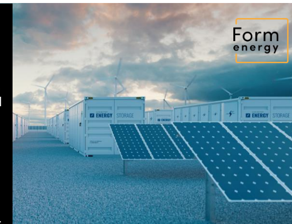
Energy Tech - Batteries
