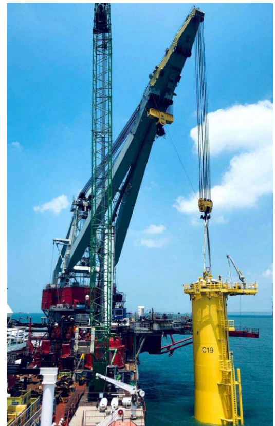
The last Transition Piece being installed
