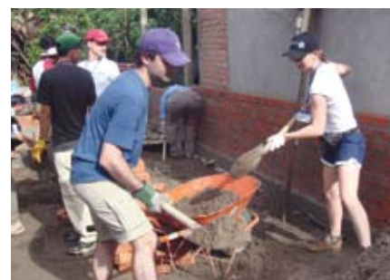
Carinda Harris shovels cement at the work site.
